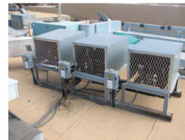
Kitchen refrigerator compressors. The R-22 refrigerant complies with EAp3, but not with EAc5.
